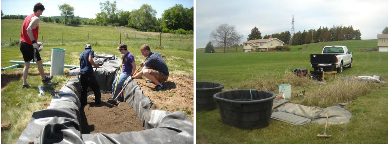
Figure 1: Filter strip excavation and membrane installation (left); planted filter strips (right)
