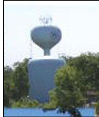
City of Waupaca water tower
