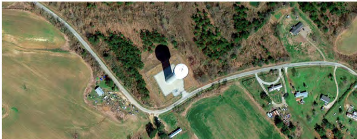
Satellite image of a portion of the Megasite of West Tennessee. (Tennessee Department of General Services.)
